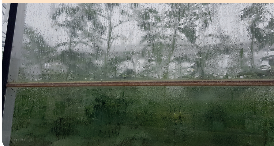
Figure 2: Large droplets of condensation forming on the glass
